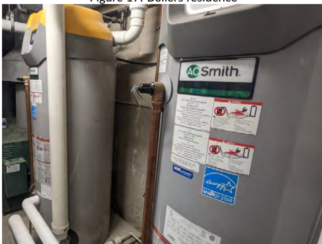
Figure 19: DHW heater
