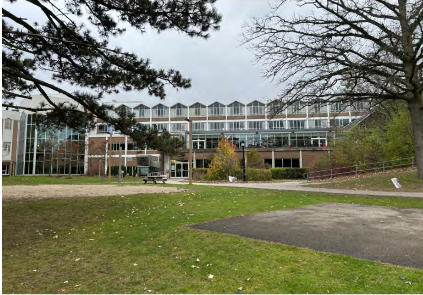
EXISTING VIEW FROM REAR OF BUILDING
