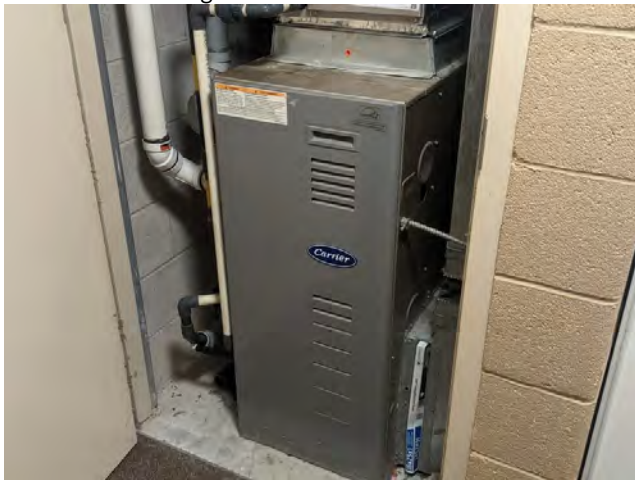
Figure 23: Furnace apartment
