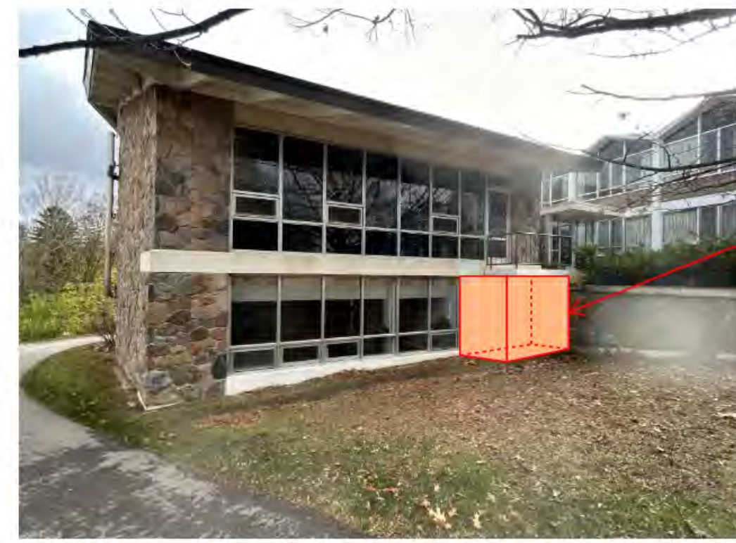
Proposed location of outdoor condensing unit AC-1. Piping to be routed to/from split chiller CH-1 as shown in Room 2431a.
