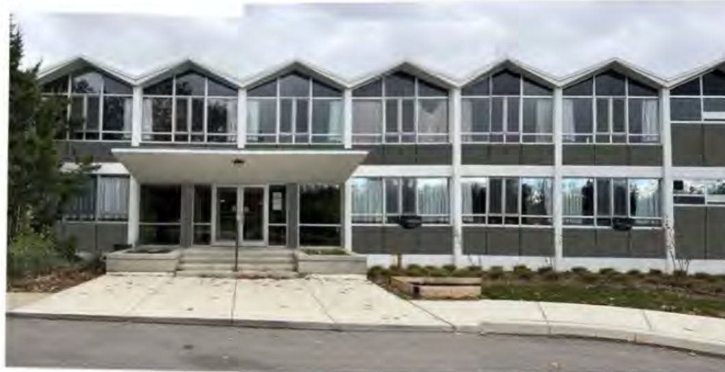
OPTION 2: FIBER CEMENT PANEL INFILL
