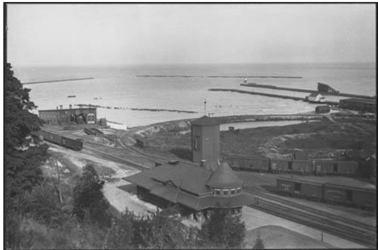
Figure 7: CRP Station in 1916 Note the piers constructed in the 1870s and the north and south breakwaters added in the early 1900s. (Library and Archives of Canada)
