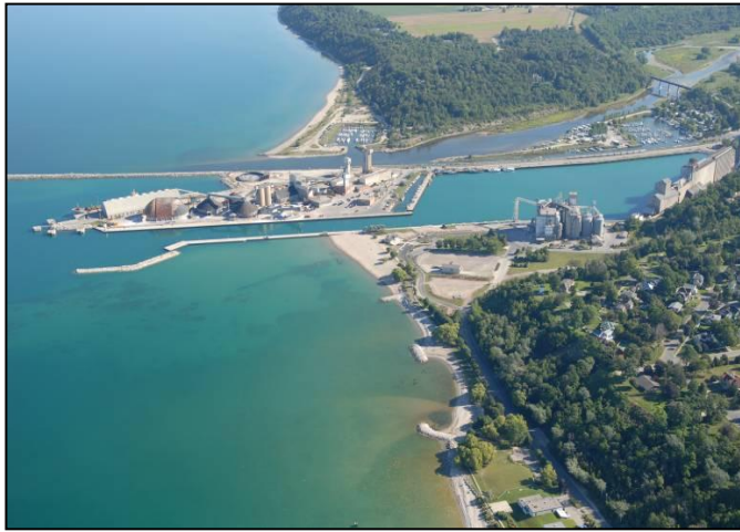
Figure 5: Aerial View of Goderich Harbour 2006 (Maitland Conservation Authority, 2006)
