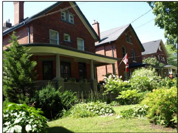
Figure 3: Well maintained and preserved buildings in Cobourg East.
