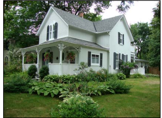
Figure 3: An example of well maintained residential building in the district.
