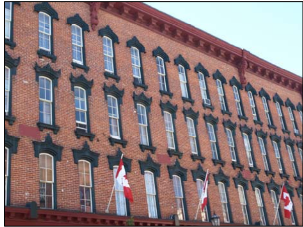
Figure 3: Example of a well maintained building
