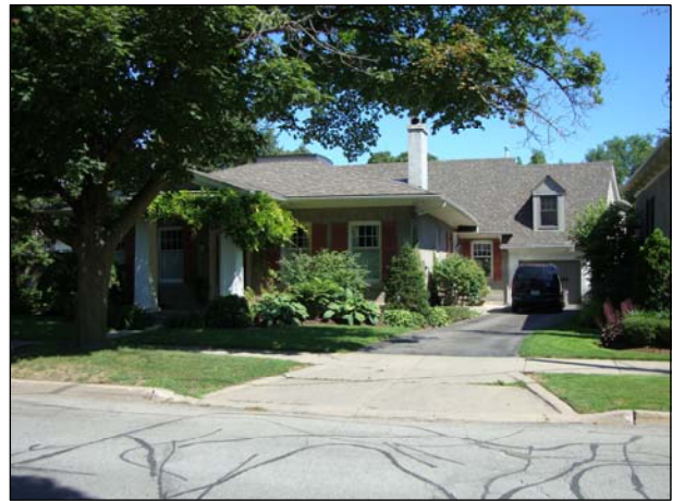
Figure 5: An example of an addition that is compatible with the character of the district.
