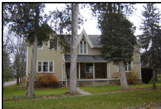
Figure 3: An example of a well maintained building
