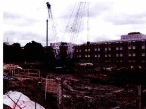
Above: Progress as of October 3rd, 2008
