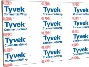
Step 2 Install water barrier and make a vertical incision halfway through window cavity.
