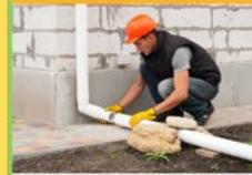
Downspouts help drain rain water from your roof to the ground. Disconnecting downspouts and diverting them away (6 feet) from your home's foundation can reduce the risk of basement flooding.
