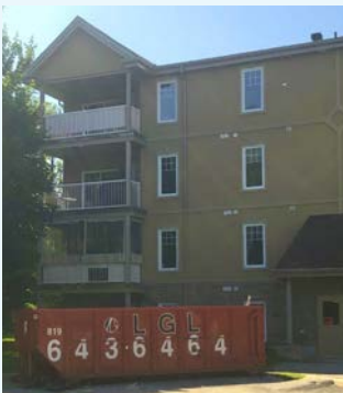
Figure 3: A 16-unit condominium in Gatineau is condemned and slated for demolition after the spring 2019 floods.
