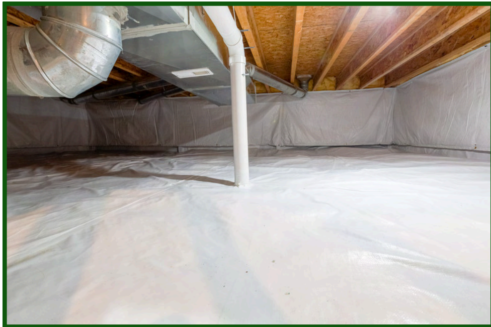
Above: Vapour barrier installed over a crawlspace ( Grandbrothers, n.d. via Getty Images/iStockphoto ).
