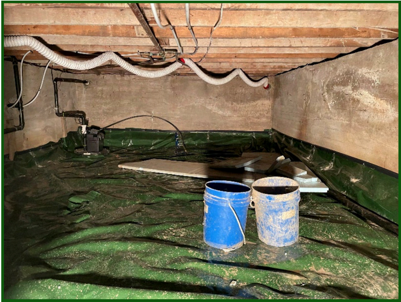
Above: Vapour barrier installed over a crawlspace that has been correctly sealed (Photo courtesy of Clean Foundation ).
