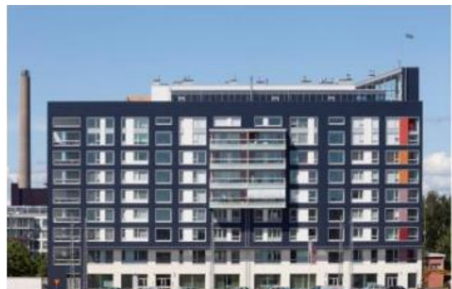
Figure 11 Casa Malta cohousing building, Helsinki
