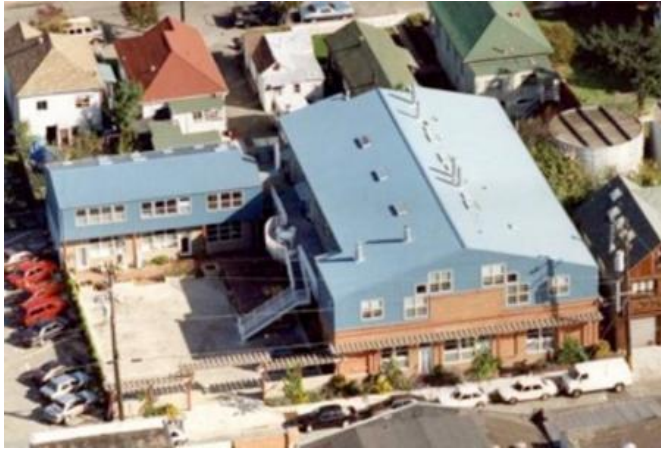
Figure 12 Doyle street cohousing community in Emeryville
