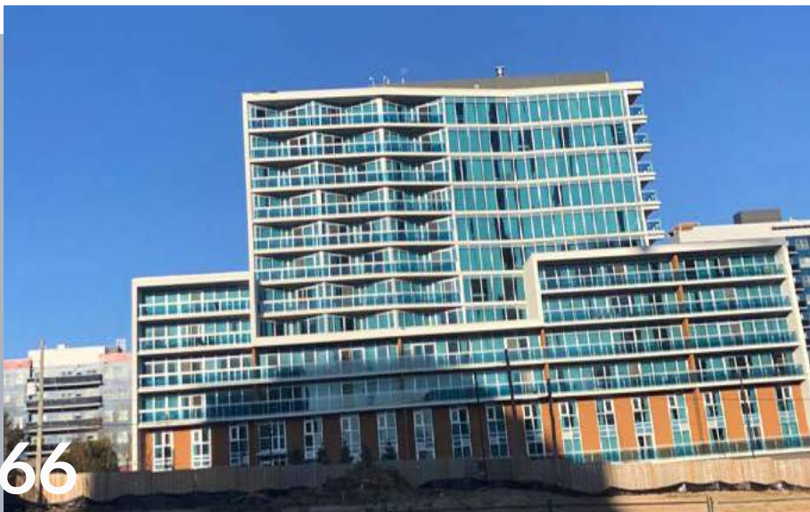
View of 255 Sunview Street
