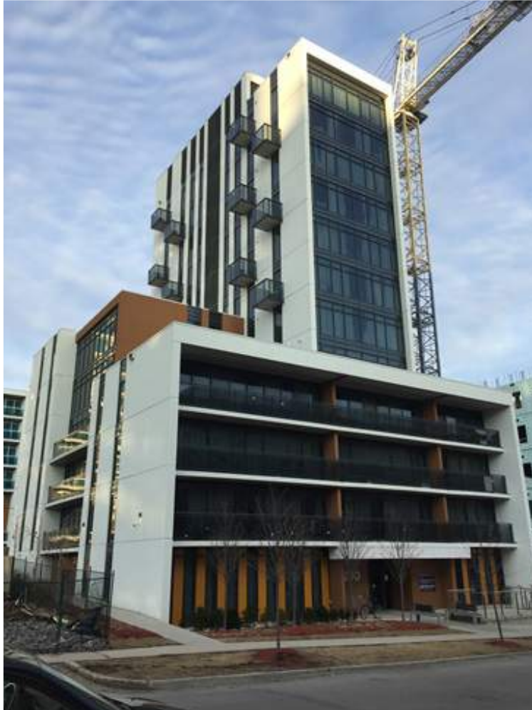
Mid-rise apartment example: 250 Lester Street, 12-storeys
