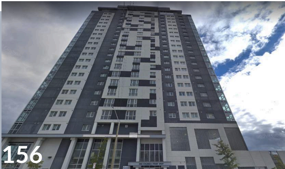
View of 1 Columbia Street West
