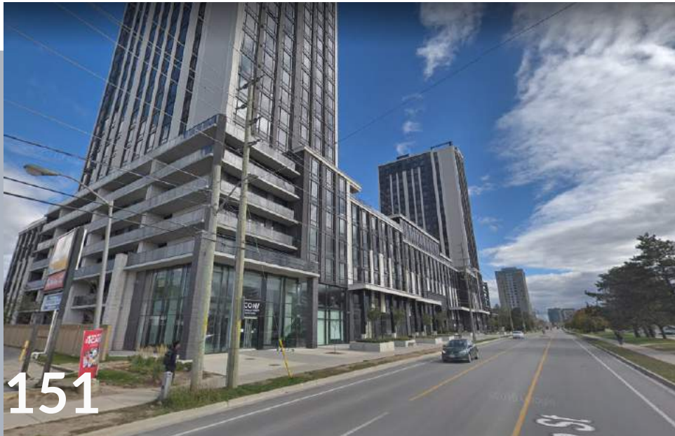
View of Phillip Street from Columbia Street
