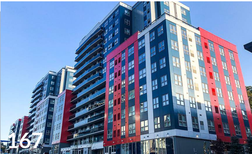
View of 250-254 Sunview Street
