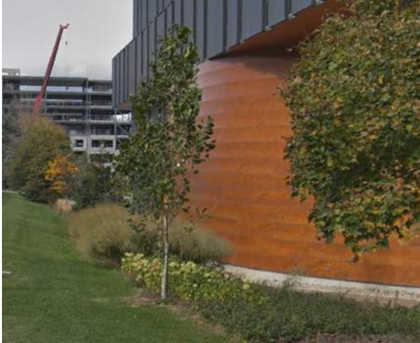
Figure 24: Stones, soil, and vegetation at the base of Lazaridis Hall (75 University Avenue) that provide stormwater infiltration
