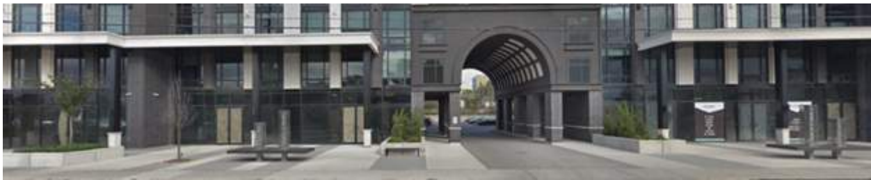
Figure 22: Impervious surfaces at 300 Phillip Street
