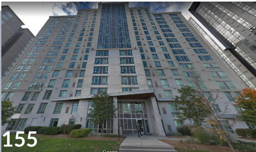
View of 333 King Street
