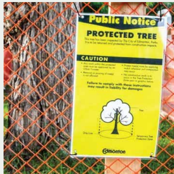
Tree Protection during Construction (CBC Edmonton, 2017)
