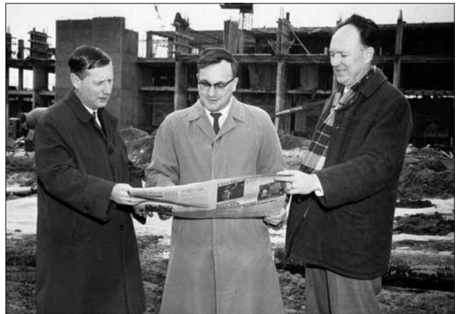
Dean Sprott and Professors Ken Fryer and Arthur Beaumont reading a newspaper ( The Coryphaeus or The Chevron ?) while standing in front of the construction site for the MC building. Photo courtesy of Chris Redmond.
