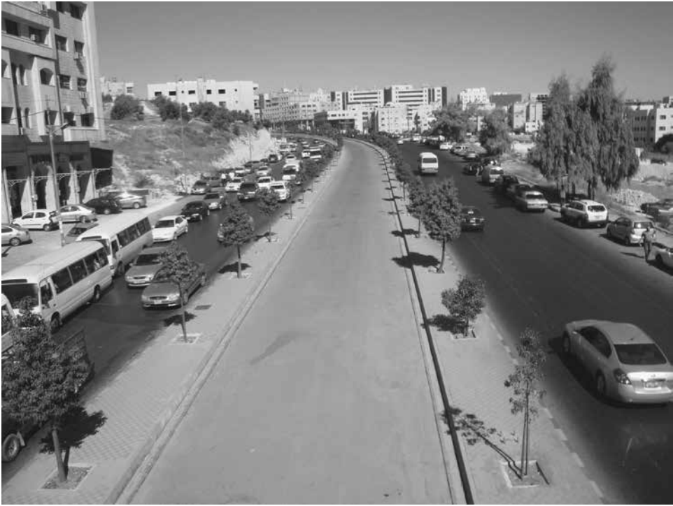
Figure 3.3 The lanes dedicated to the BRT along the University Street (Shari' al-Jami'a) have been standing unused since the halting of the project in July 2011
