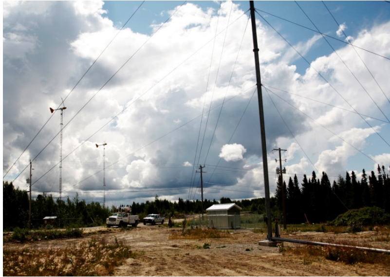
Figure 4. Small WTs installed at Kasabonika Lake First Nation, Ontario. Tilt-up towers are a feasible option to install and maintain the WTs with locally available resources.
