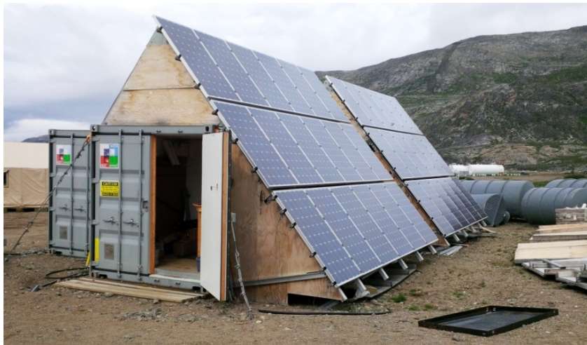
Figure 3. Solar PV system installed at the remote Torngat Mountains National Park base camp, Labrador (photo courtesy of Oliver Johnson). Similar small solar PV systems have been successfully installed in Canada's N&RCs.
