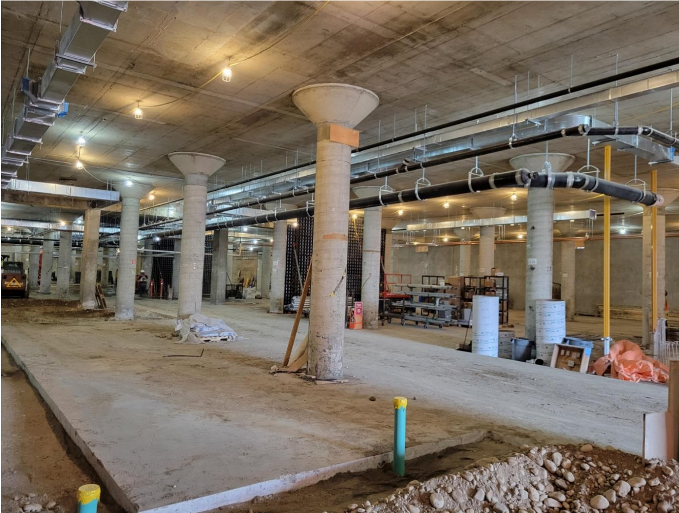
Photo below – construction progress at Innovation Arena, Kitchener Campus
