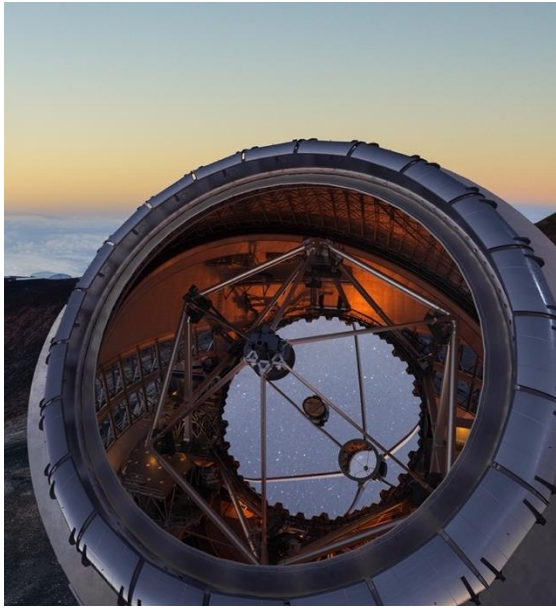
Figure 5: The 30-m primary mirror is seen through the opening in the Calotte dome, a unique design by Empire Dynamic Structures Ltd., a Canadian company based in Burnaby, BC.
