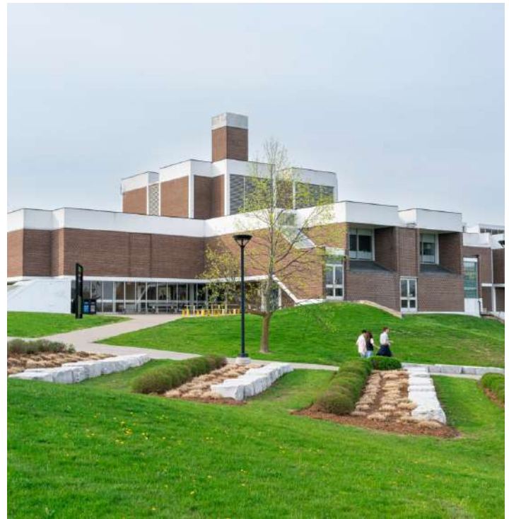
Figure 37. South Campus Hall is a building with high deferred maintenance. The site has strong potential to contain a new district energy nodal plant, an innovation hub, ancillary services, alumni spaces, an art gallery, and classrooms.
