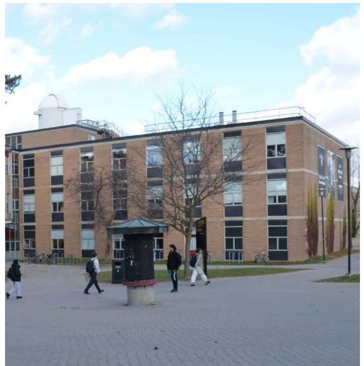
Figure 35. The Physics building is recommended for minor renovation.
