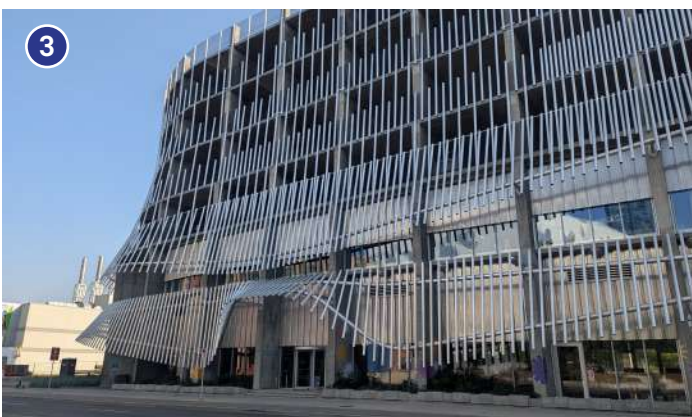
Figure 160. Structured parking with screening
