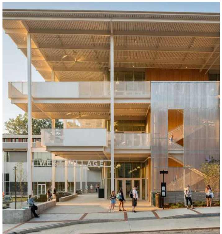
Figure 48. Covered walkways and enhanced visibility create a safer and more enjoyable transit experience (Community Hub at Georgia Institute of Technology)
