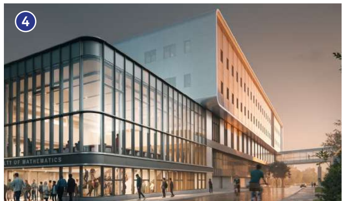
Figure 140. Math 4 framing William Tutte Way (Moriyama Teshima Architects)
