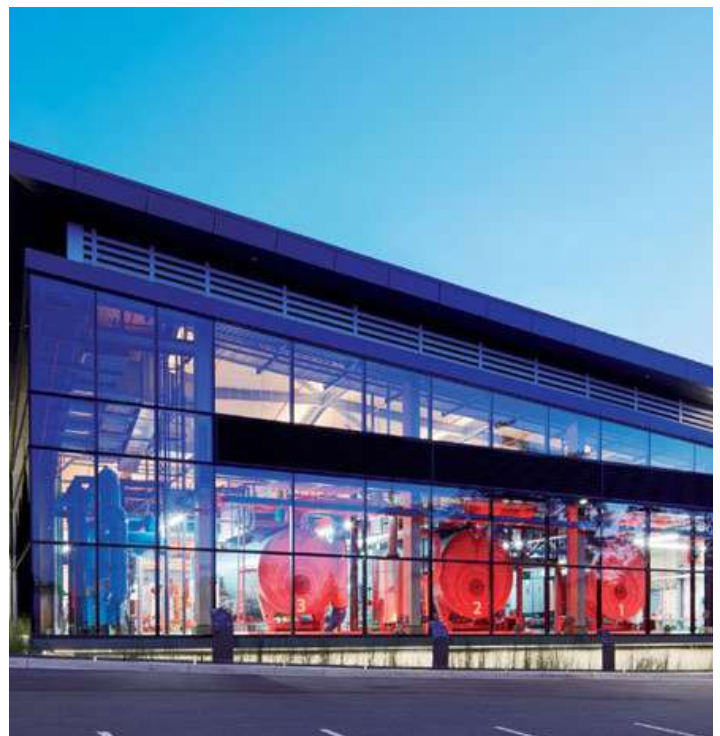
Figure 38. The district energy plant building at the University of Victoria features rainwater harvesting, the use of structural wood, and high-efficiency glazing, demonstrating the University's commitment to sustainability.
