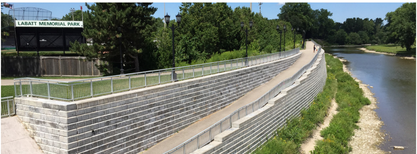
Above: West London Dyke Reconstruction
