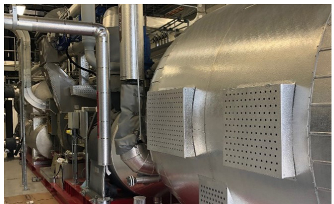
Above left: On the left is a rendering of the Organic Rankine Cycle system before its arrival and installation in London. Above right: the Organic Rankine Cycle system is pictured in 2021 now in operation.
