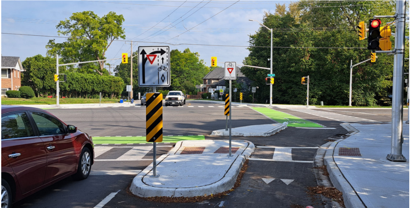
Above: One of seven new protected intersections recently added throughout the city
