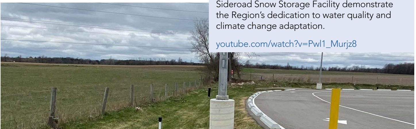
Looks can be deceiving – The Charleston Sideroad Snow Storage Facility.
