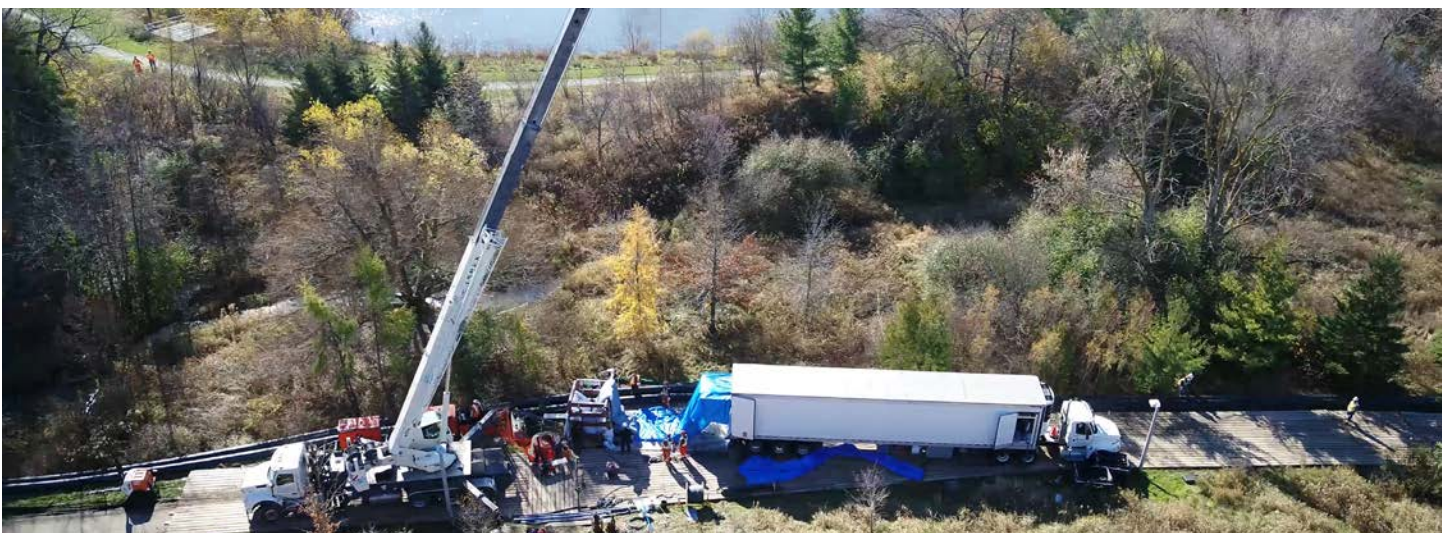
Valve chamber is on its way
