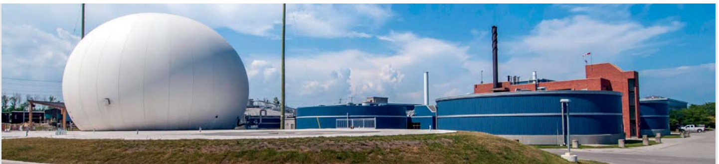
Cogeneration at the Clarkson Water Resource Recovery Facility.
