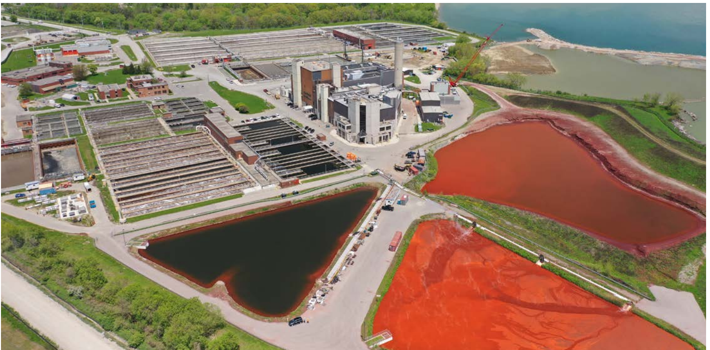
Ash ponds at the GE Booth Resource Recovery Facility.
