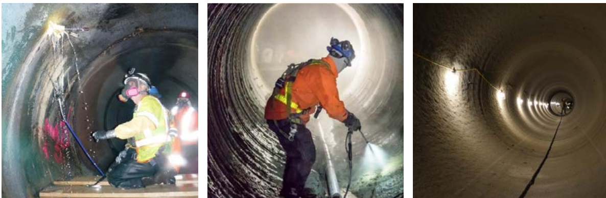
Photos left to right: Grouting, Cleaning, Sewer after completion
