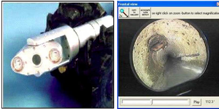
Fig. 1. CCTV camera and internal inspection image of buried pipelines.
