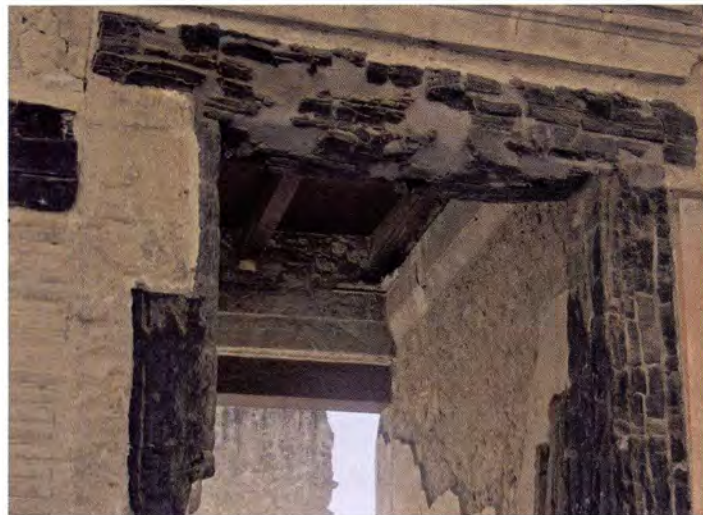
Figure 6: Herculaneum; one of the massive doorways. The beams above the gateway are charred from the base surge.
