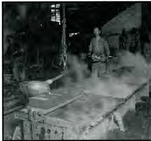
Pouring molten copper into ingot molds, Calumet — Hekla Mines, Calumet, Michigan.
