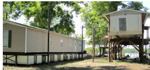
In Louisiana, after the spring 2011 flood. Amphibious house on left is undamaged. Note waterline on elevated house on right.
