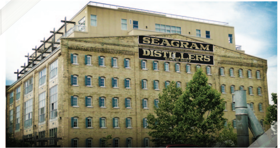
Seagram Distillery buildings now converted to condominiums
