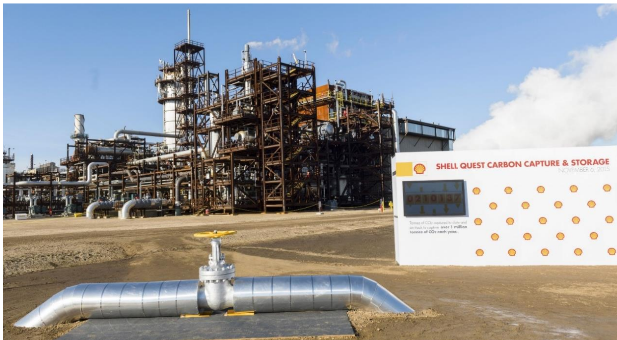
Figure 4: Quest Amine Absorption Unit, Scotford Refinery (courtesy Shell Canada)
