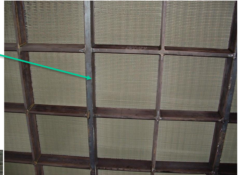
Upstream Side View
