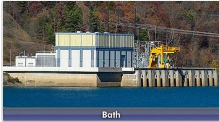
Pumped Storage Hydro
