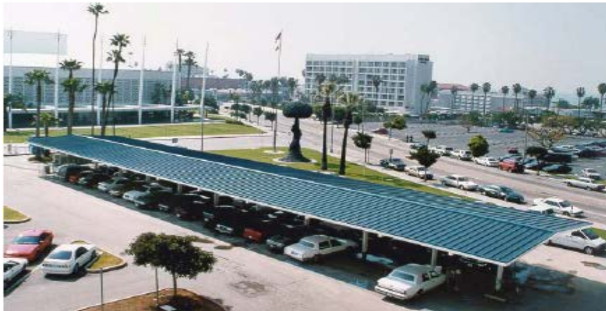
30 kW EV Charging Shade Structure
