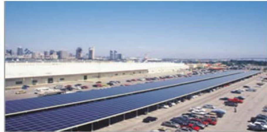
300 kW EV Charging
