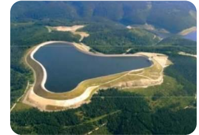
Source: Schluchsee plant
