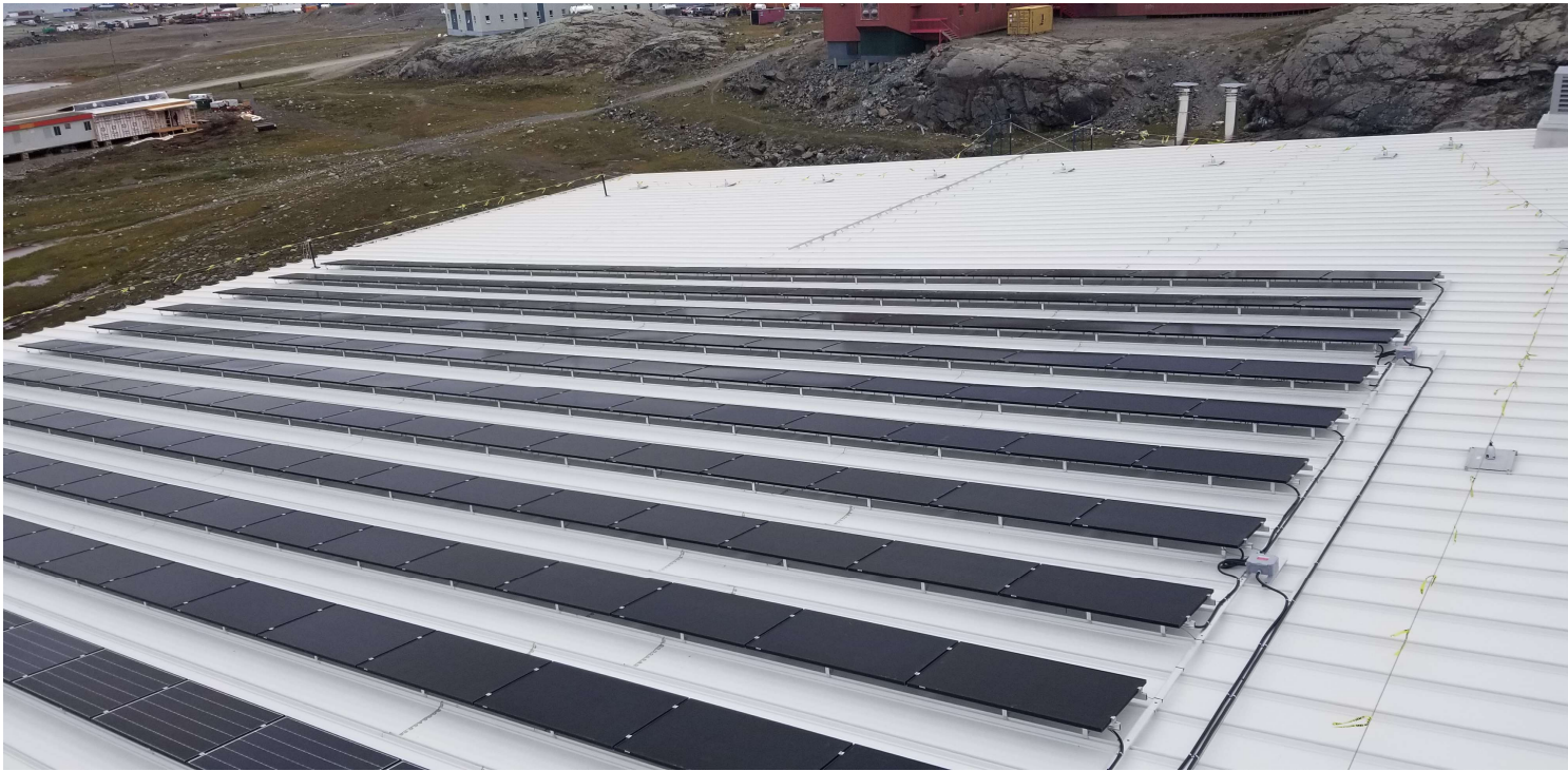
Rooftop installation with S-5 clamps on standing seam metal roof
