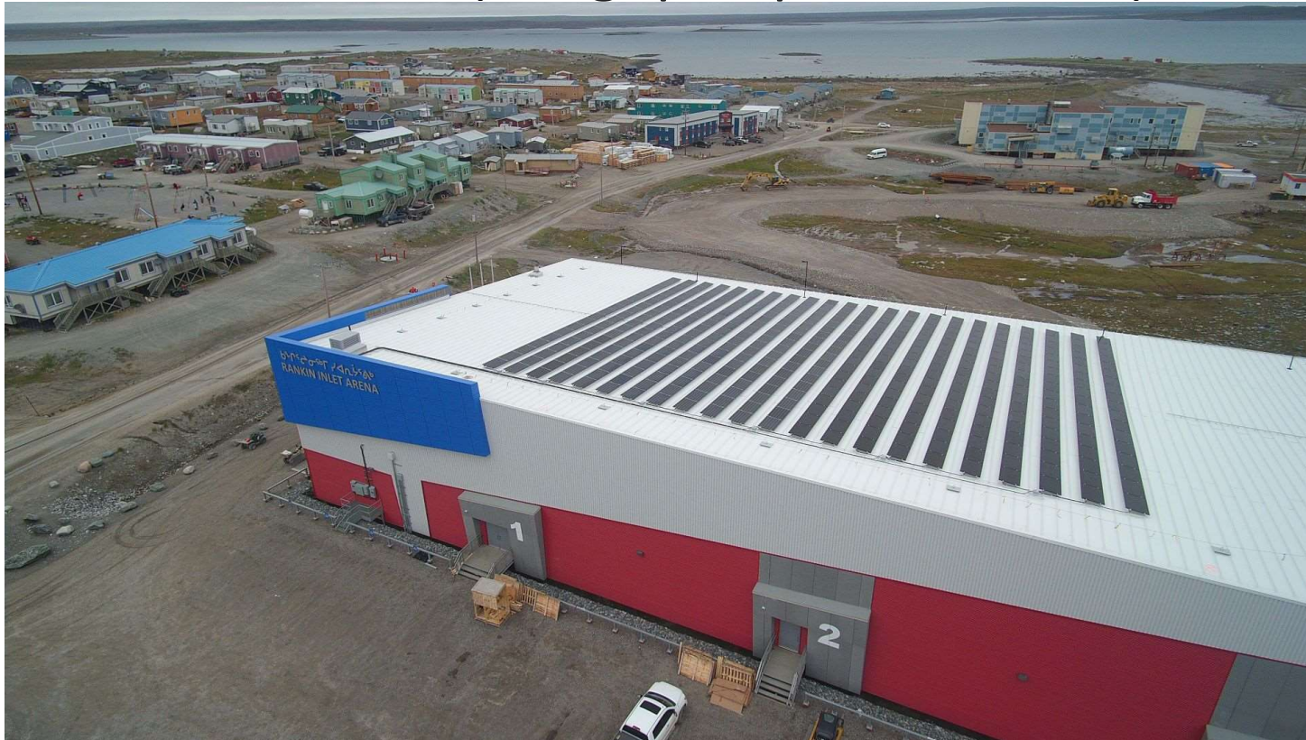
126.72 kW DC and 110 kW AC solar PV system
