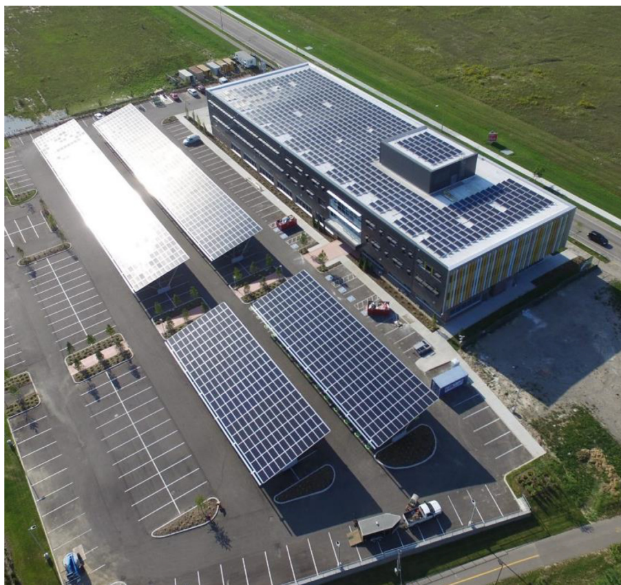
Fig. 1. Case study building exterior showing parking lot and roof solar PV systems, image from (11).
