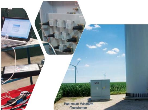
Dielectric Spectroscopic Analysis of Windfarm Transformer
